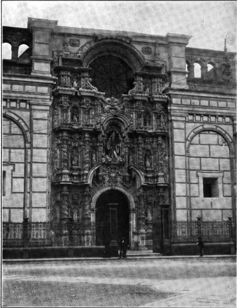
Façade of San Augustin Church, Lima
